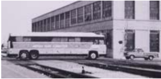
An MC-8 crosses Santa Fe tracks at the Bakersfield station in California.
